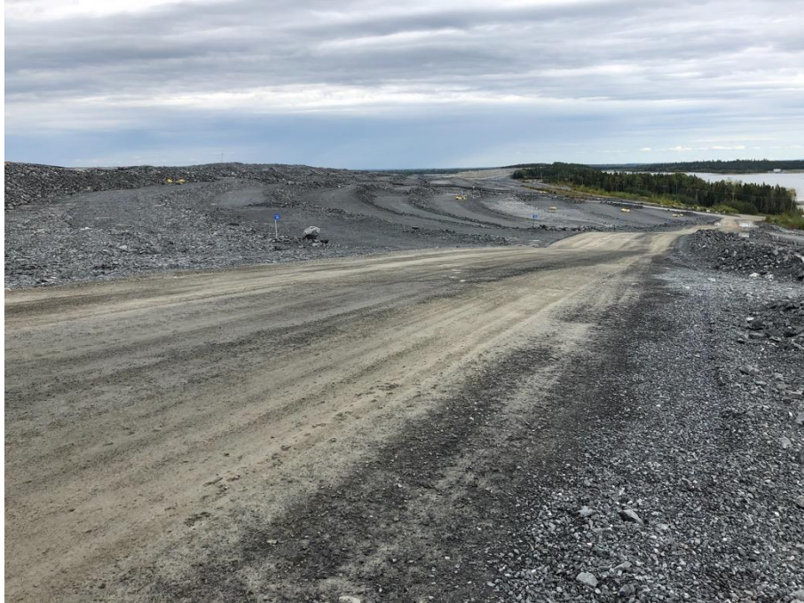
Figure 3.1: Mine haul roads at Canadian Malartic Mine (2019); the wearing course was constructed using crushed waste rocks and the base course was constructed using uncrushed waste rocks.
