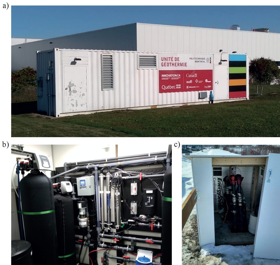
Figure 2. Mobile geothermal laboratory used during this study, (a) general outside view, (b) groundwater treatment unit and (c) view of the SCW head.
