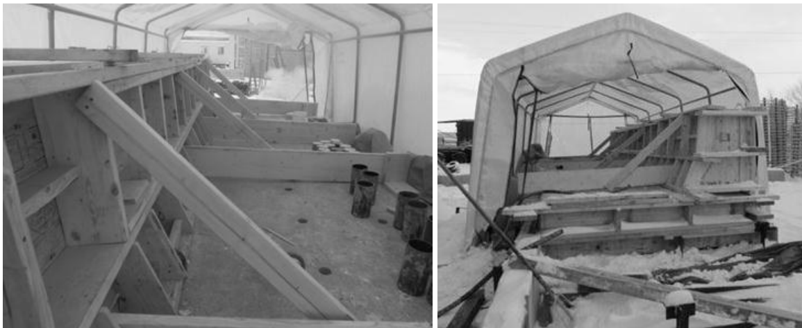
Figure 5-12: Formwork Assembly and Fixation, Cast-in-place Barrier
