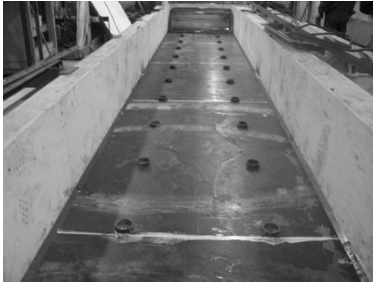
Figure 5-7: Block Formwork
