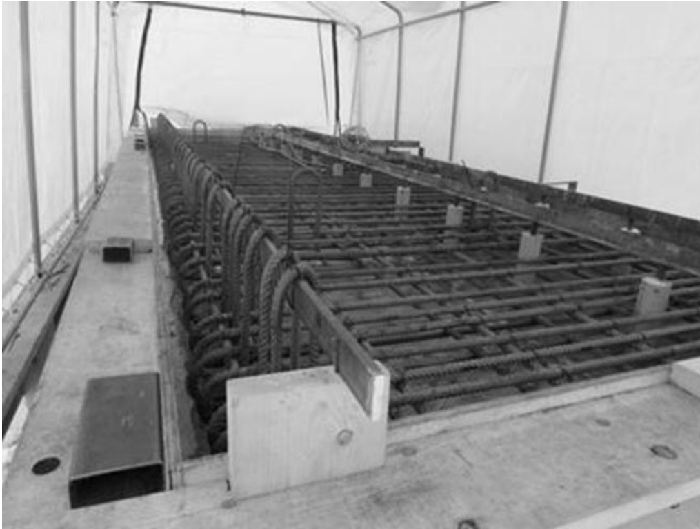
Figure 5-9: Slab Reinforcement and Anchor Support
