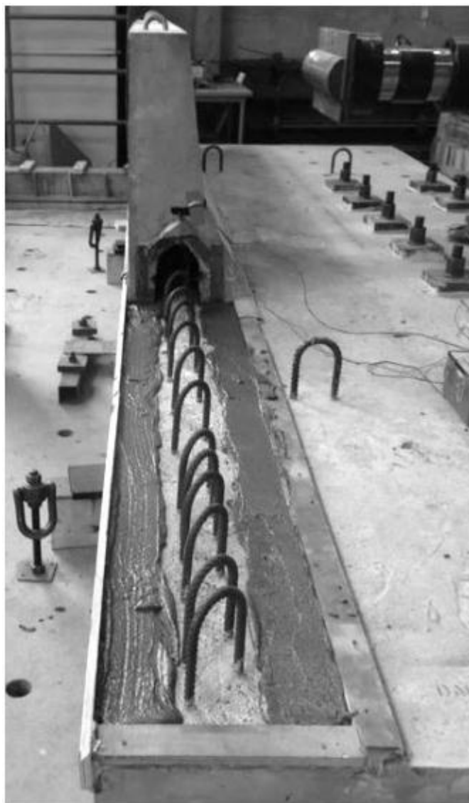
Figure 5-26: Mortar Bed for Precast Barriers
