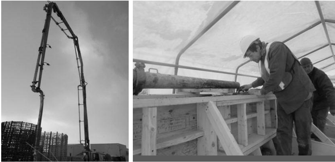
Figure 5-13: Barrier Pour with Industrial Pump
