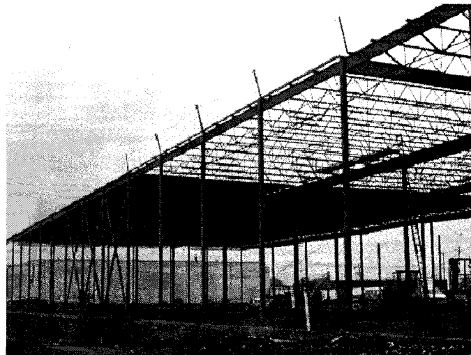
Figure 1.1 Typical single-storey steel structure
