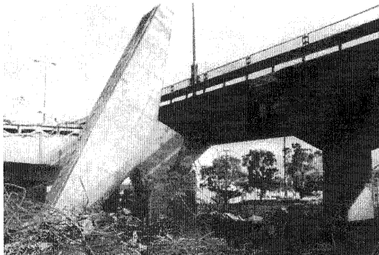
Figure 2.3 – Rupture en cisaillement-flexion (Priestley et al., 1996)
