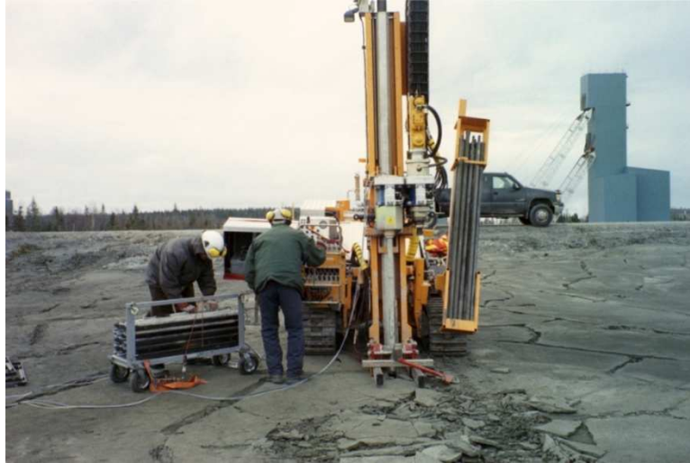
Figure 3-3 - Operation of the CPT rig on the impoundment.
