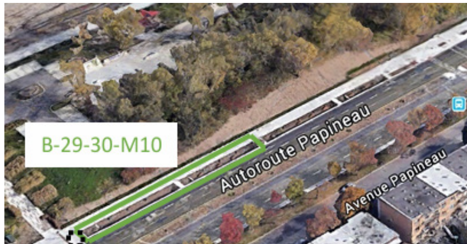
Figure 1 Example of a bioretention basin (B-29-30-M10) located along Papineau Avenue, Montréal.
