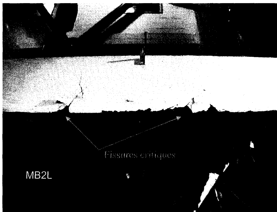
Figure 7.12: MB2L – Fissures critiques
