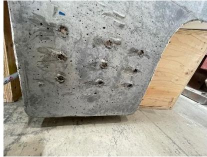
Figure 5.28 – Extremity face of girder G2 showing tendon slippage after the shear test
