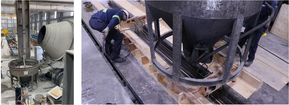
Figure 4.7 – HPFRC transfer from the truck to the bucket and from the bucket to the formwork
