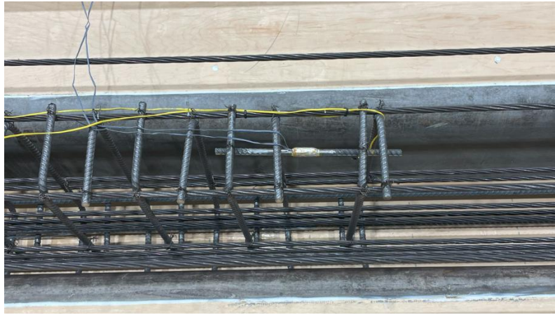
Figure 4.8 – Sensor cable layout
