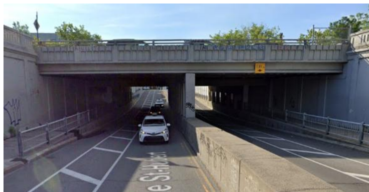
Figure 3.1 - Example of an underpass bridge in Montreal
