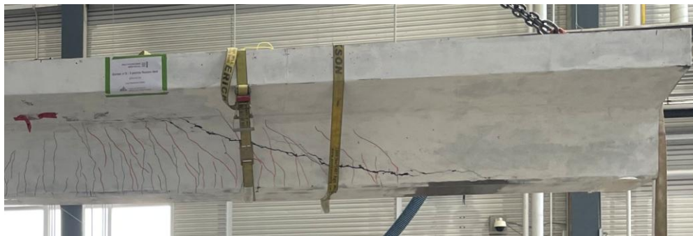
Figure 4.25 – Cracking pattern of girder G2
