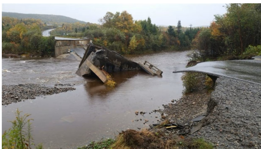
FIGURE 1.4 Rupture du pont de St. Alban's
