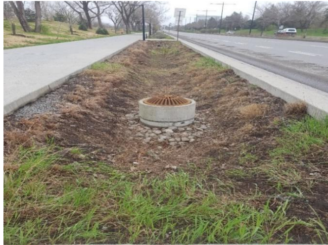
Figure 3.1 Bioretention basin at the Papineau project, photo taken during the May 02, 2024 visit
