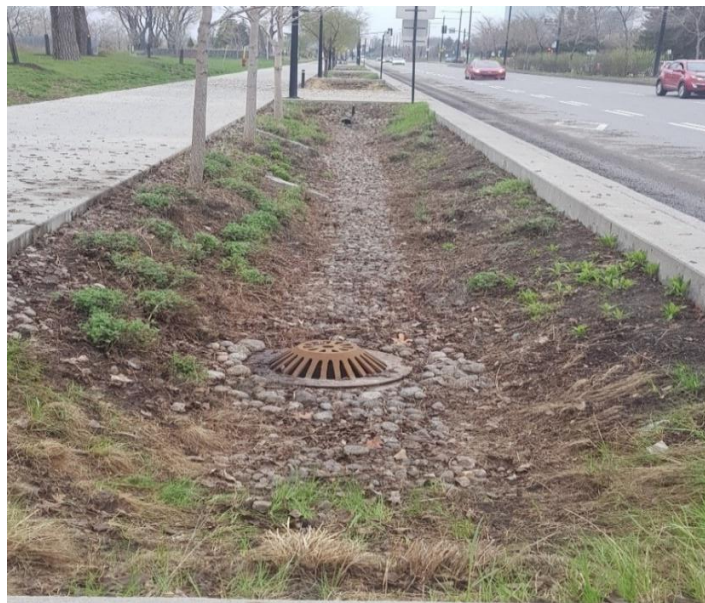
Figure 5.2 Vegetated retention basin for the Papineau project
