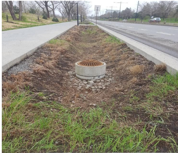
Figure 5.1 Bioretention basin of the Papineau project
