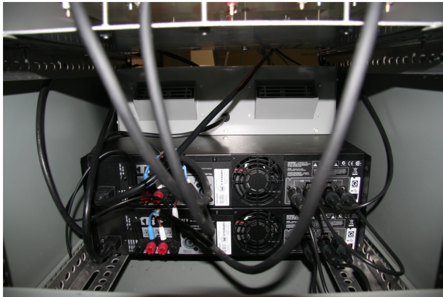
Figure C.4: Power amplifier connection
