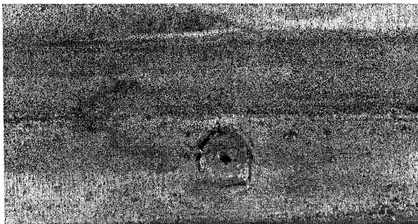
Figure 4.133. Example of weld quality at non-side-lap connections (G21)
