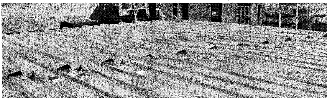
Figure 4.69. Sheet deformation at overlapped joint (Gridline 11)
