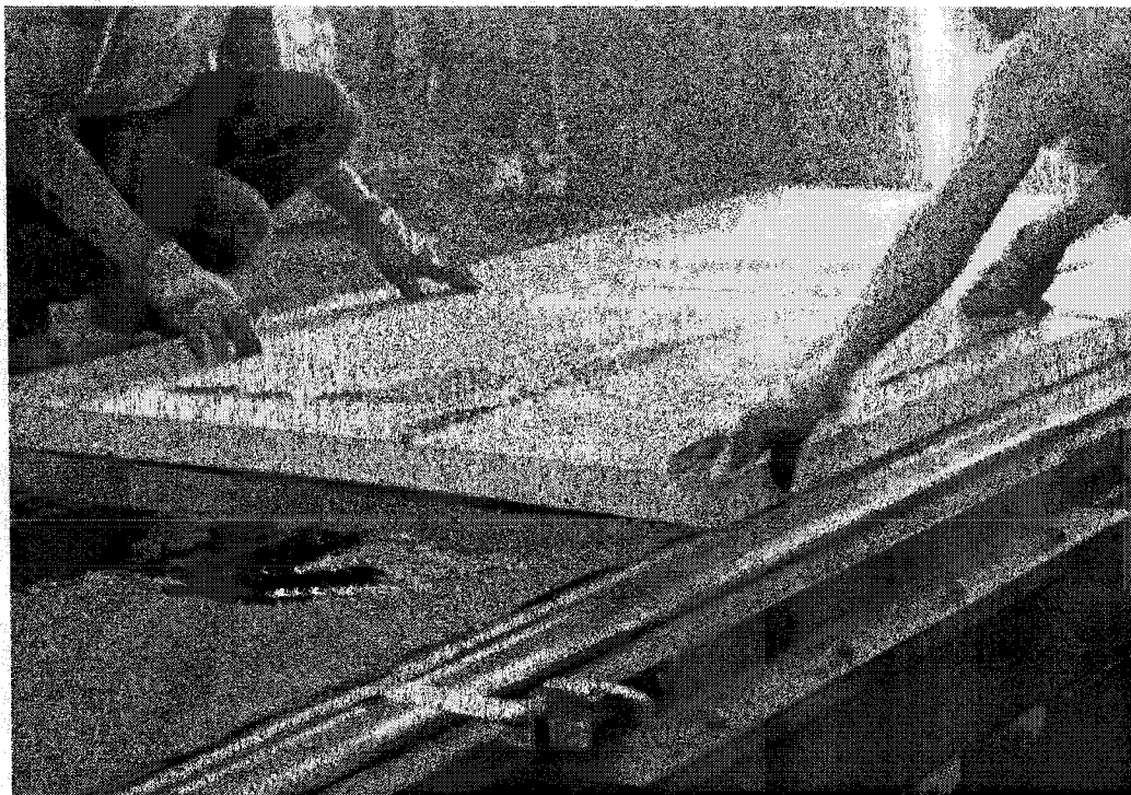
Figure 4.25. Installation of ISO insulation board
