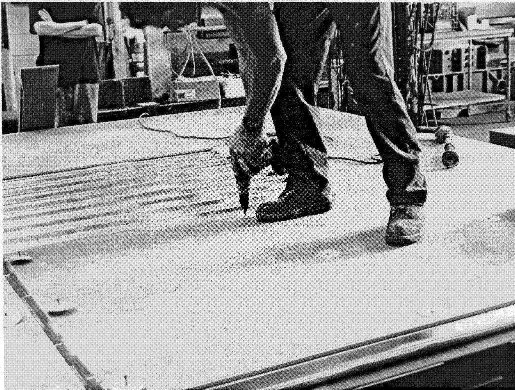
Figure 3.8. Installation of gypsum board on steel deck
