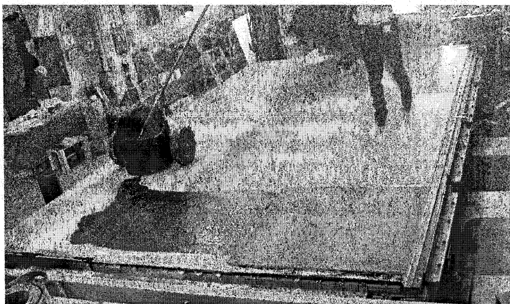
Figure 4.26. Installation of wood fibreboard above ISO insulation layer
