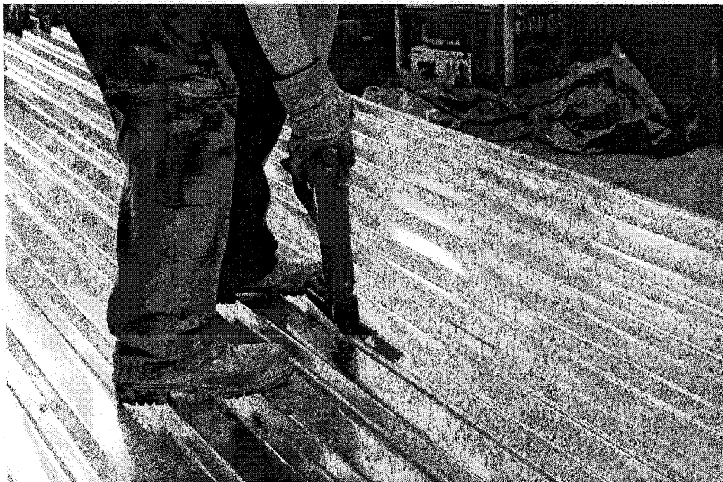
Figure 4.18. The installation of powder actuated nails
