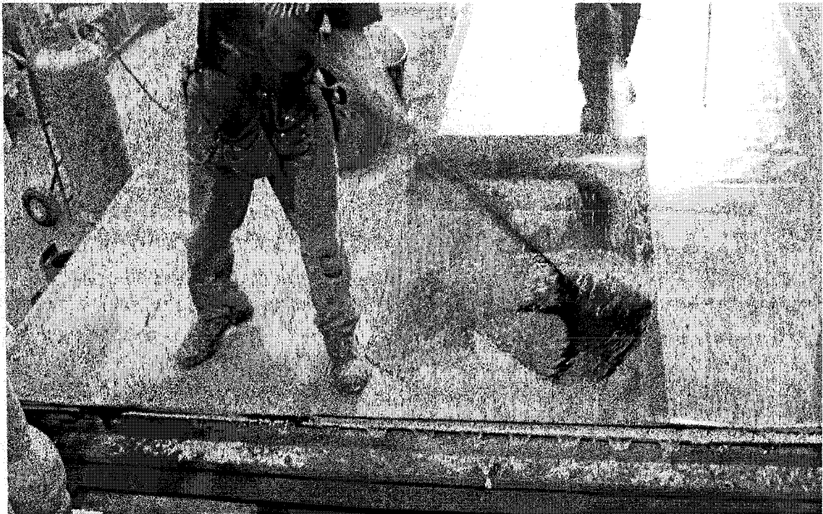
Figure 4.28. Installation of SBS base sheet by hot bitumen and flame torch
