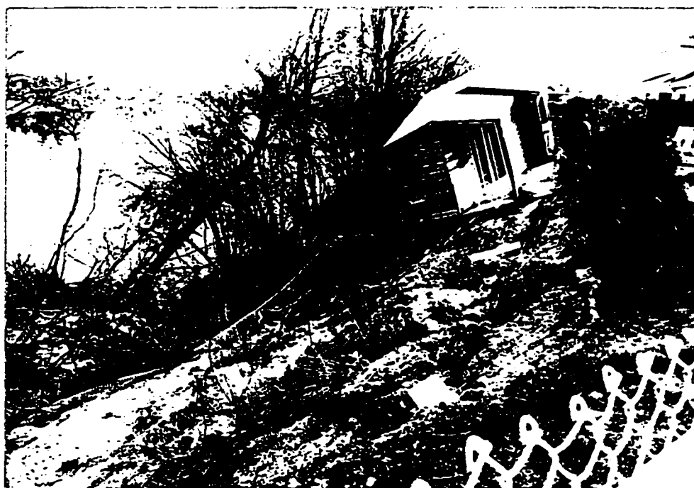
Fig. 6-3 Effect of latest landslide on residential buildings
