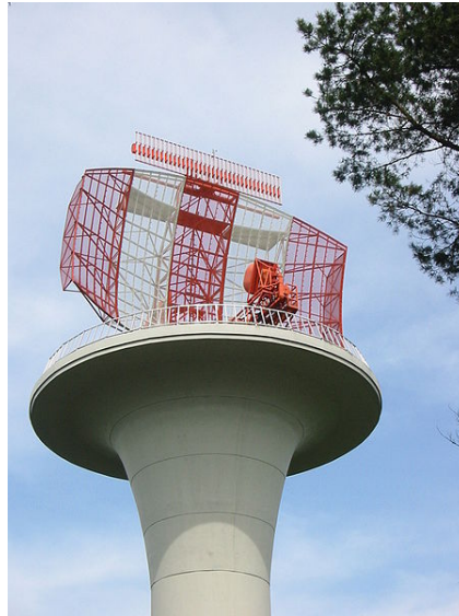
Figure 5.1 Radar antenna on the Deister river close to Hanover, Germany. The parabolic antenna is the primary radar and the rectangular one above it is the secondary radar. The secondary radar interrogates the transponder on the aircraft, which sends back a coded signal identifying the craft and giving its altitude (reproduced from [173]).
