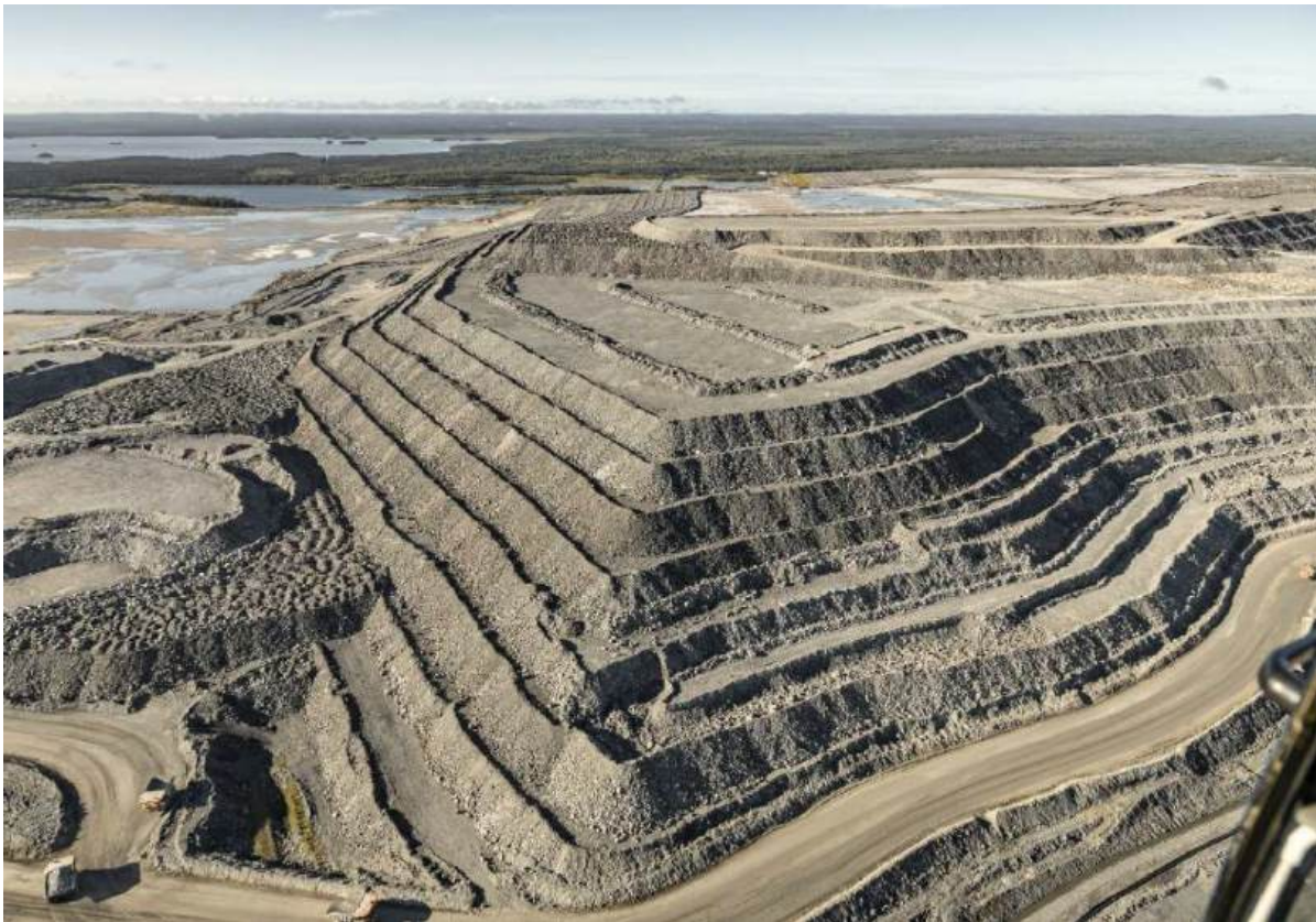
Figure 2.12 WRP constructed with benches at Canadian Malartic Mine after Aubertin et al. (2021).
