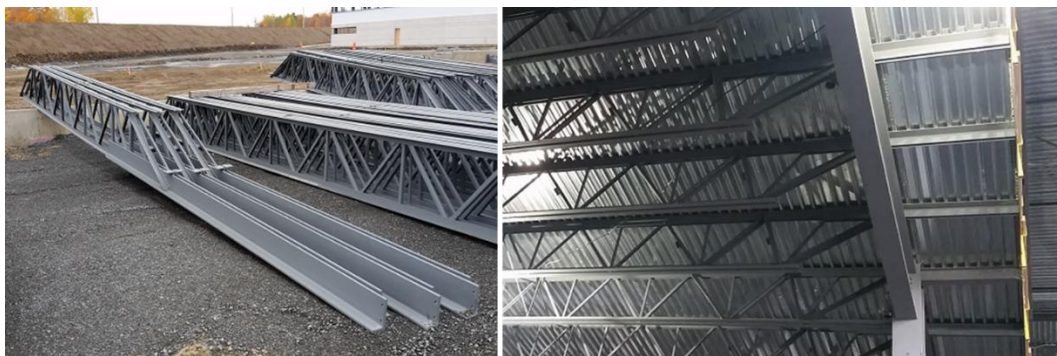
Figure 4-2: Steel joists with top chord extensions for a cantilevered floor in an industrial building: prior to erection (Left) and after installation (Right)
