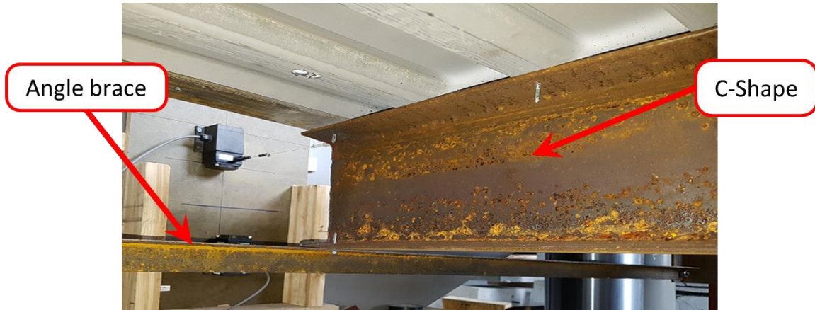
Figure 4-9: Steel angle used to provide point bracing at the tip of the bottom flange of the C-shaped top chord extension.
