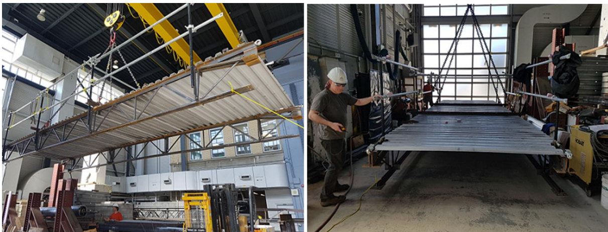
Figure 4-6: Lifting operation of the "exterior joists - steel deck - guardrail" assembly.
