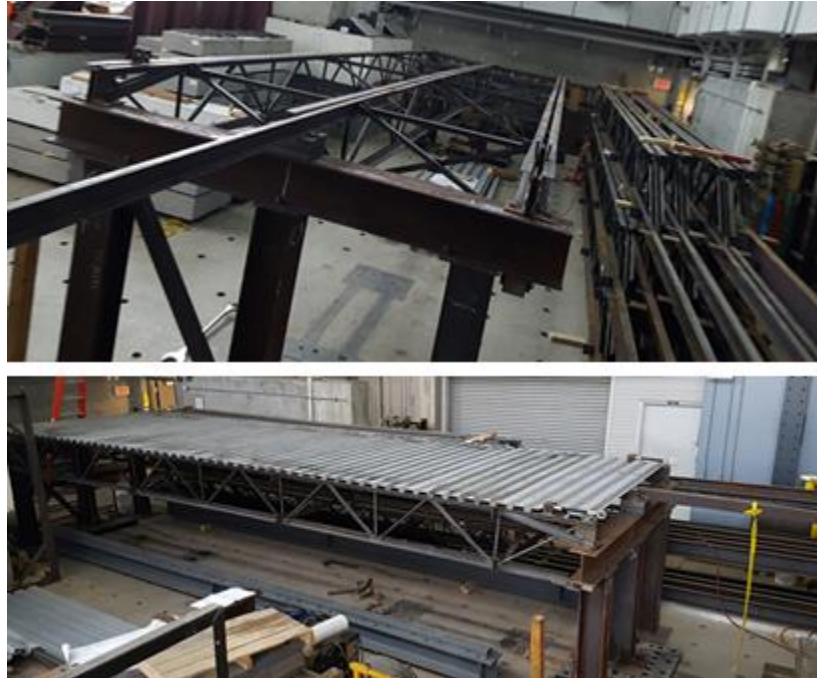
Figure 4-5: Vertical support and lateral bracing conditions for the steel joist specimen.
