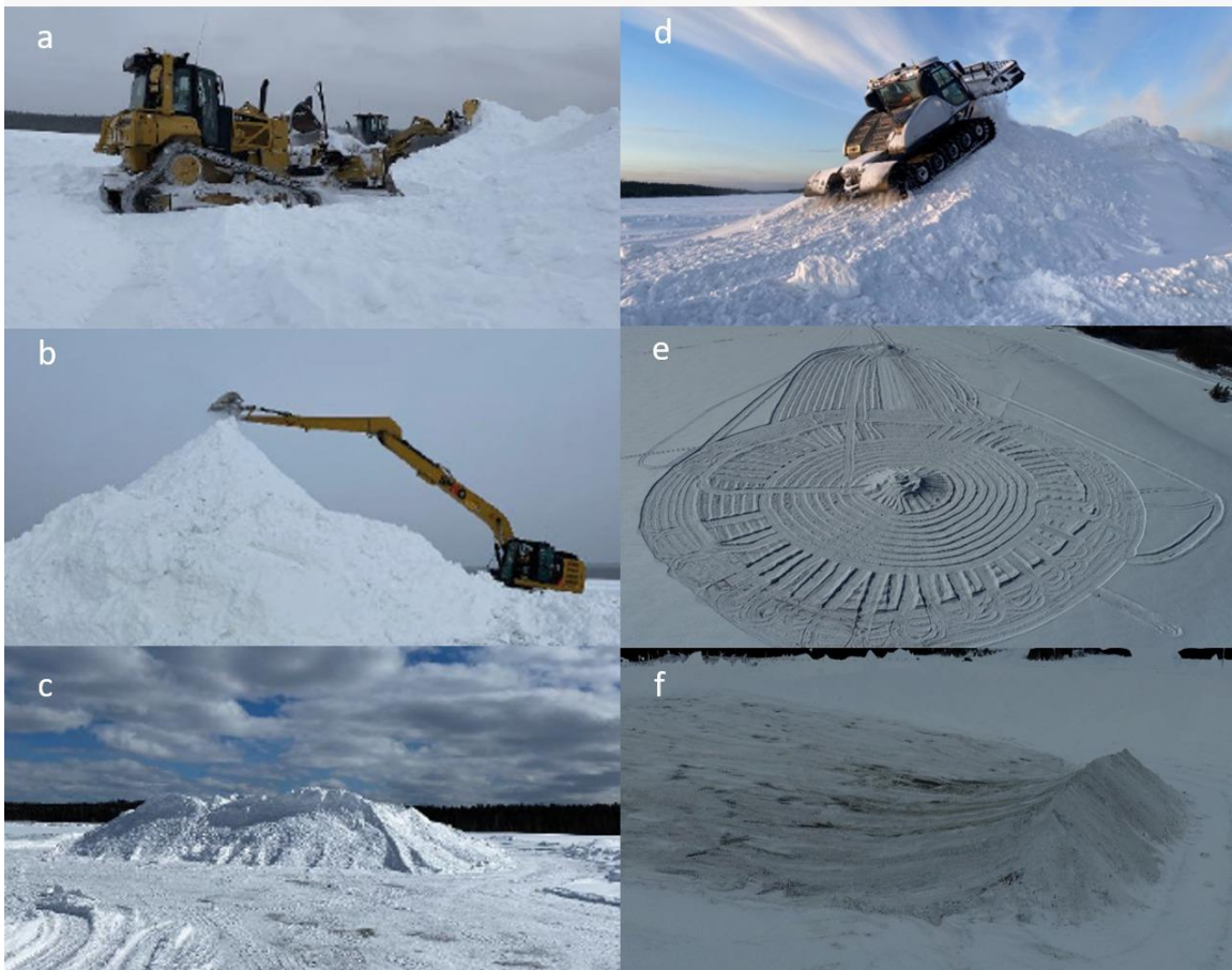
Figure 3.1 (a) Crawler dozer and wheel loaders used for the construction of SMPs in 2022; (b) hydraulic excavator lifting the conic SMP in 2022 and (c) final profile of the cubic SMP in 2022; (d) snow groomer used for the construction of SMP in 2023; (e) final profile of conic SMPs as well as groomer track on the snow in 2023; and (f) final profile of the ramp-shaped SMP in 2023.
