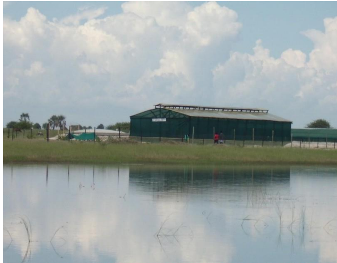
Figure 6: Floodwater harvesting pilot plant at Iipopo (Namibia)
