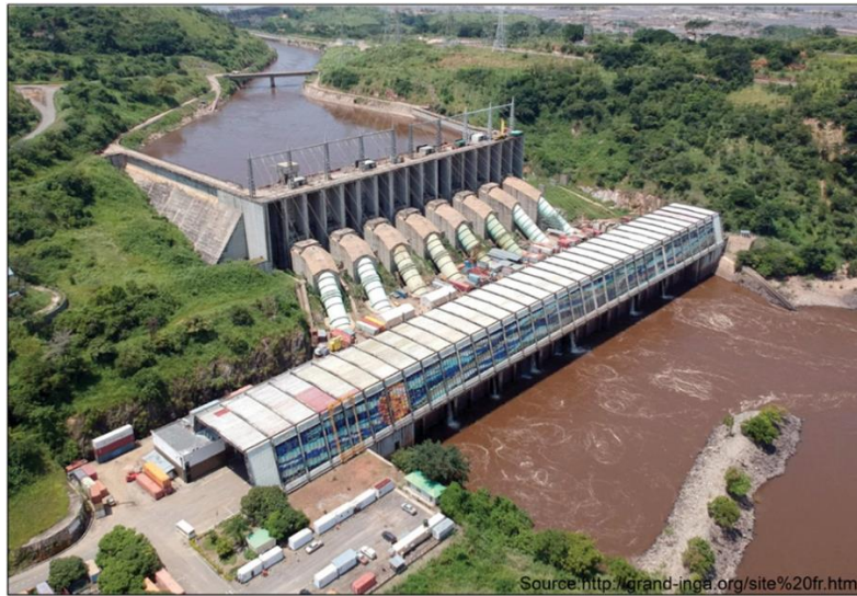
Fig. 11 View of the Inga 2 hydro plant.
