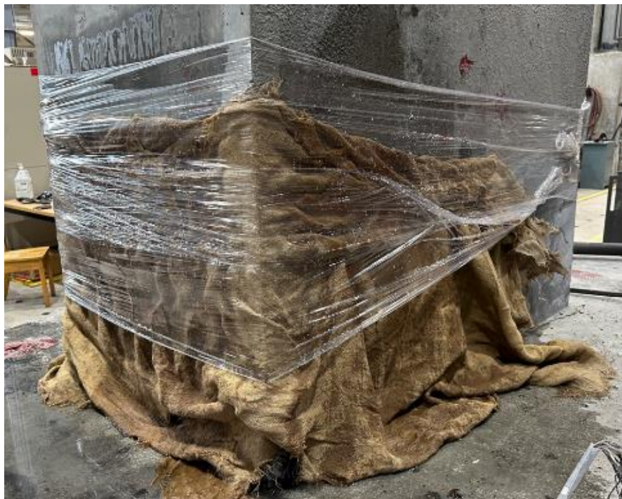
Figure 5.18 Cure humide du joint
