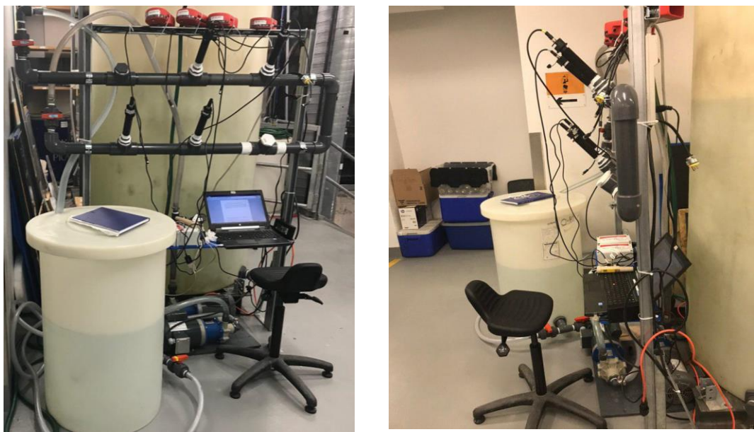
Figure 3.4 Pipe-loop used for the evaluation of the KAPTA 3000 AC4 and OT3 probes
