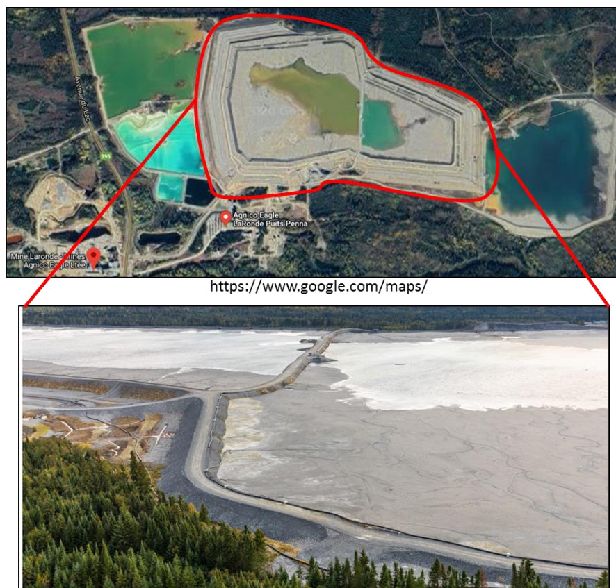
Figure 6.1 LaRonde tailings storage facility.
