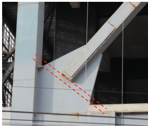
Figure 2.20 Free length and reinforcement plate. Reyes (2018)
