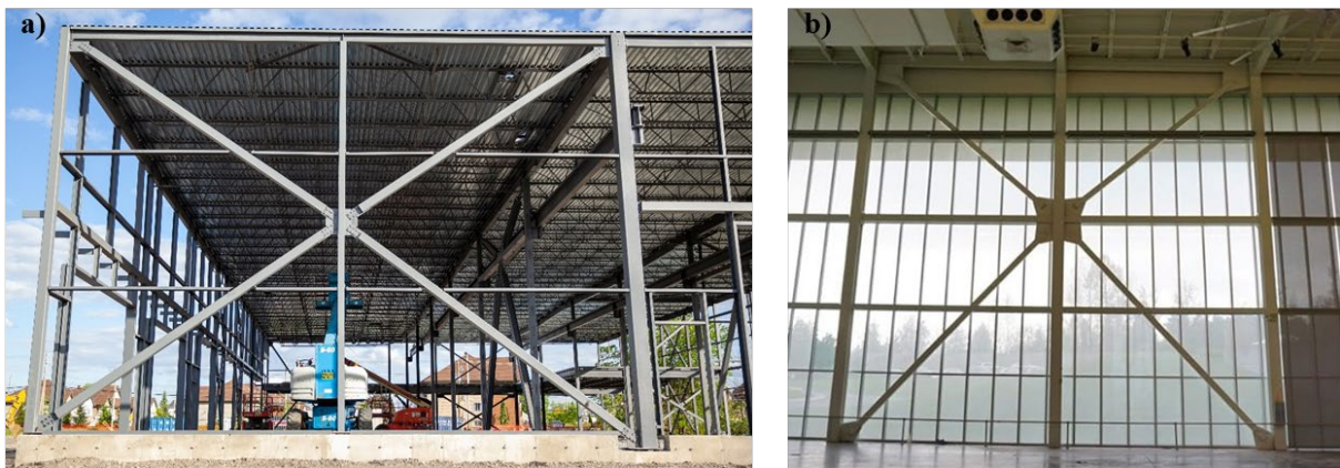
Figure 7.1 Example of two-bay X-CBFs: a) without intermediate strut; and b) with intermediate strut
