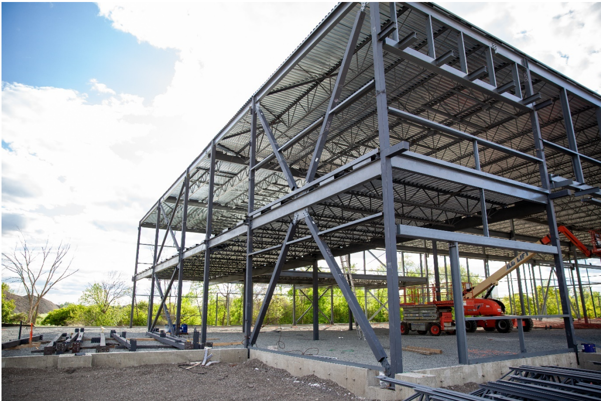
Figure 2.1 Example of an inverted-V steel CBF in Varennes, Qc
