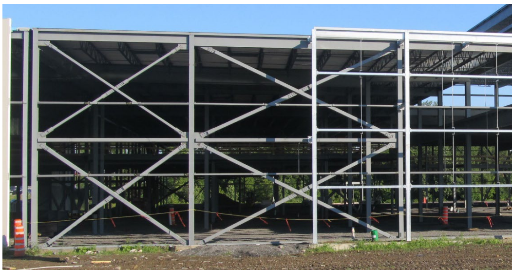
Figure 1.2 Example of a two-bay two-tiered CBF
