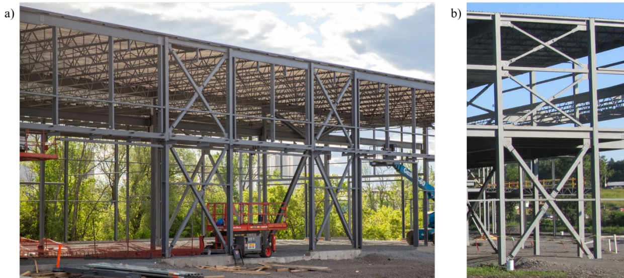
Figure 1.1 Examples of MT-CBFs: a) construction of an industrial building using two-tiered concentrically braced frames in Varennes, QC; and b) example of a multi-storey MT-CBF
