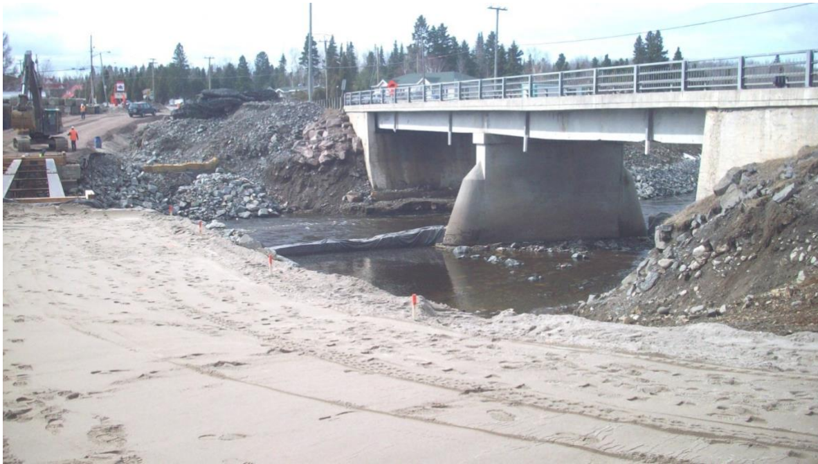
Figure 6-5 Pibrac Bridge: for high discharges, the pillar is an obstruction to the flow, increasing the water level upstream. Note the cofferdam installed to limit suspended sediment release
