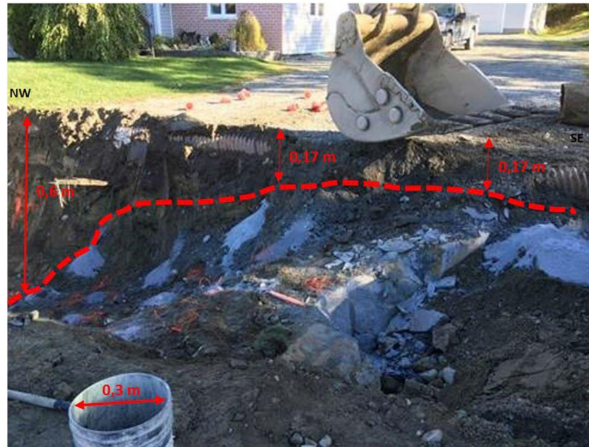
Figure 3.14 : Image made during excavations on Clericy Street, highlighting a near-surface and undulating bedrock (rhyolite).
