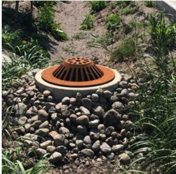
Figure 4.3 Overflow downstream drain of a bioretention basin
