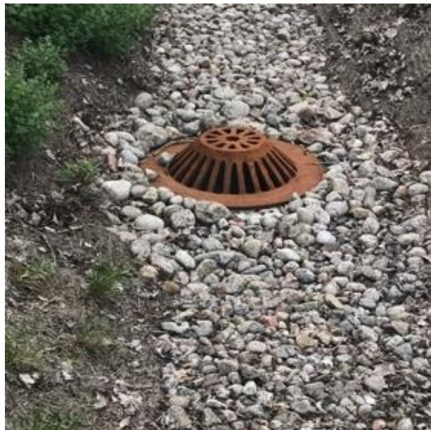
Figure 4.4 Lowered downstream drain of a vegetative swale
