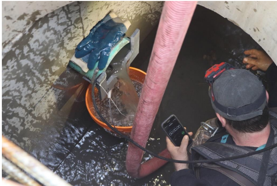
Figure B.10 A view of the set up inside the monitoring manhole
