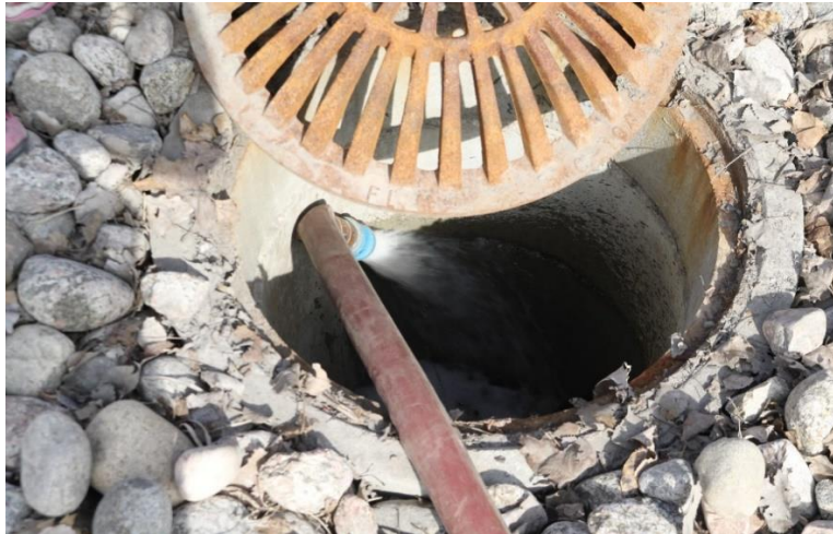
Figure B.8 Connecting the pump to the outflow point: the drain of the vegetated swale which is upstream of the weir
