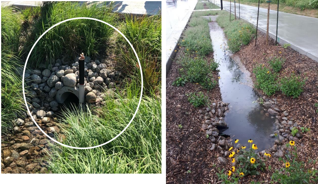
Figure 5.5 Piezometric well measuring the ponded depth of runoff stored in a bioretention cell
