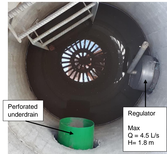
Figure 4.5 Top view inside the downstream overflow of a bioretention basin showing the regulator fitted on the conduit connecting the structure to the sewer line
