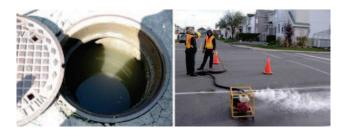
Figure 1. Flooded air-vacuum valve vault.
