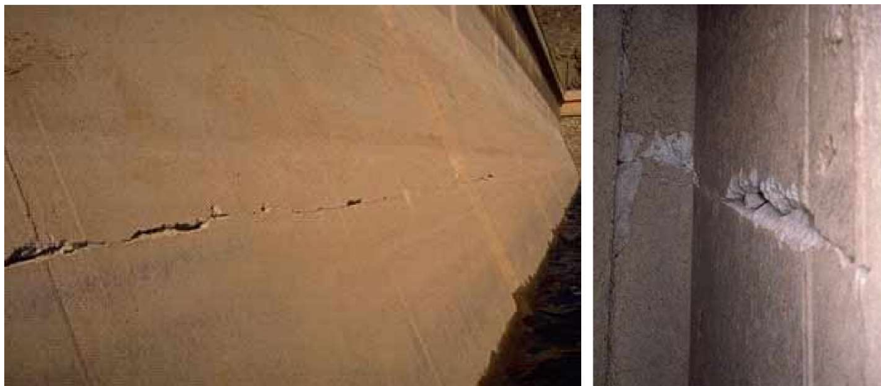
Figure 2.1 Sefid Rud buttress dam - Horizontal cracks at lift joints (Wieland and Fan, 2004)
