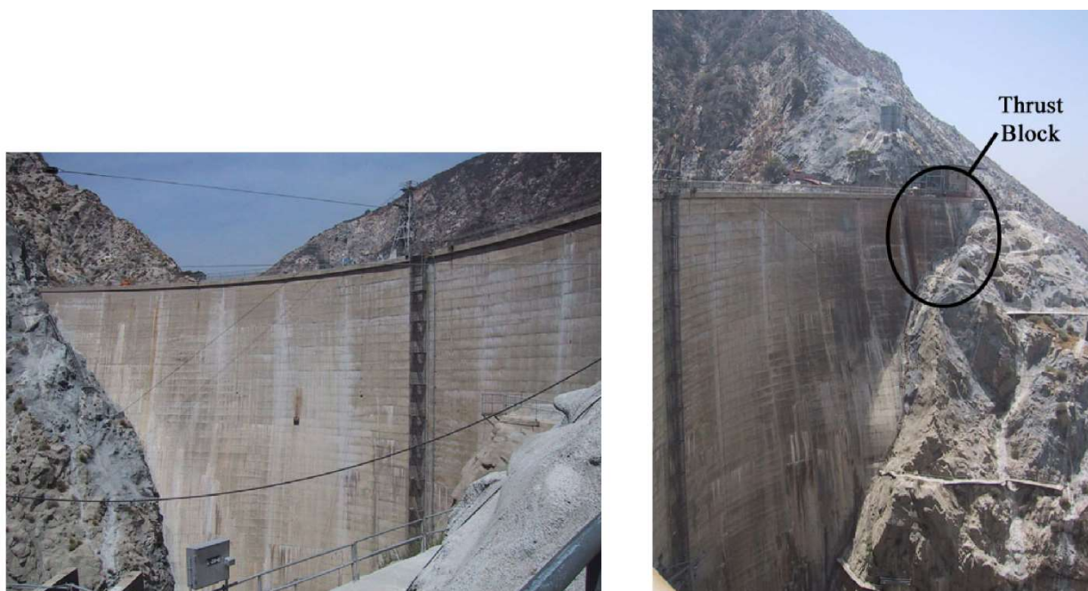
Figure 2.2 Pacoima dam – left and right abutments (Alves, 2005)
