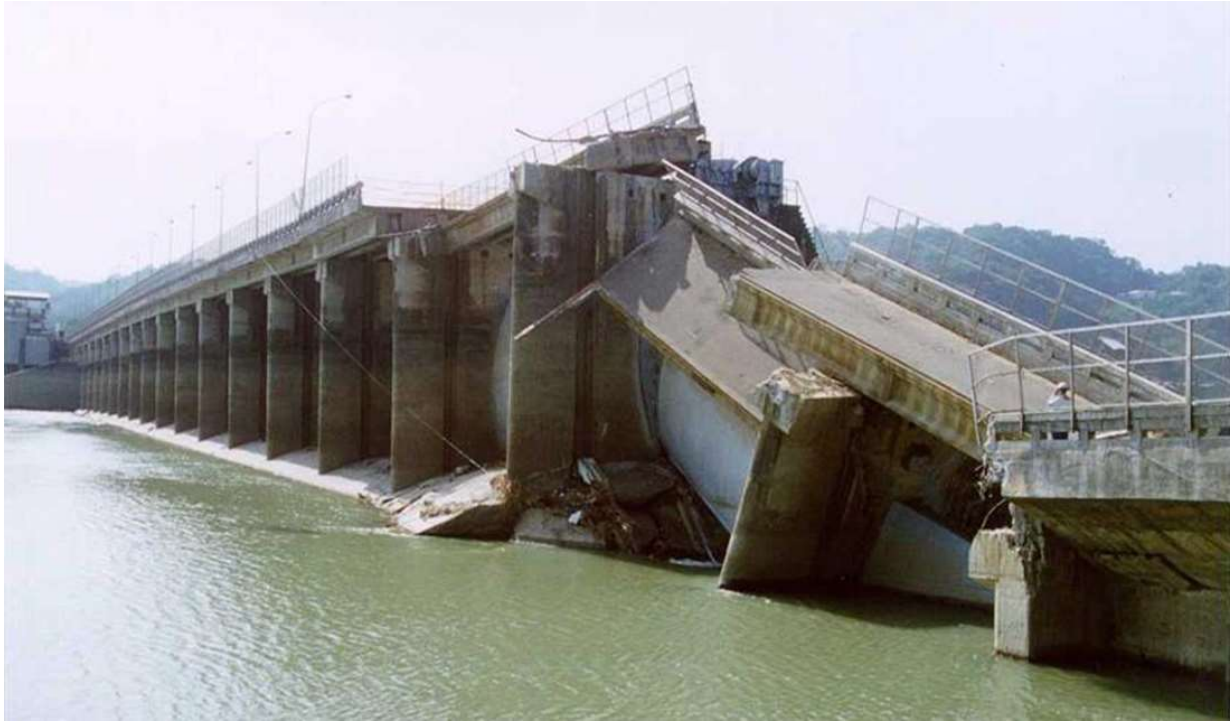
Figure 2.3 Failure of Shih-Kang dam during Chichi earthquake in Taiwan (Wieland, 2016)
