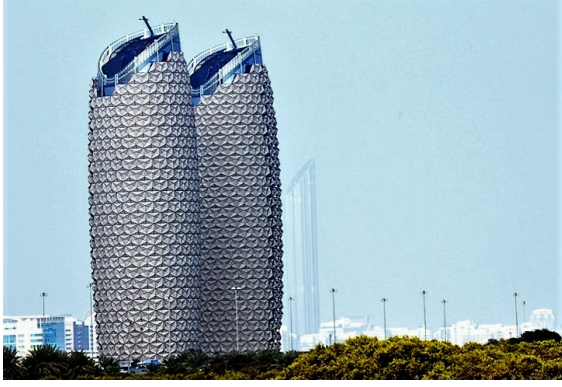
Figure 6.1 Dynamic façade, Al Bahar Headquarter, Abu-Dhabi, United Arab Emirates (Inhabitat, 2014)
