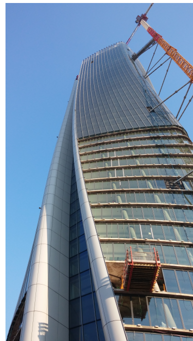
Figure 2.2 Torre Hadid during the construction of the double façade, Milano, Italy (Salerno, Ilaria. 2017)
