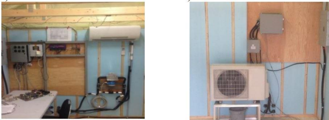
Figure 2-3: Indoor (left) and outdoor (right) unit of the VCASHP (Tardif et al. 2016)
