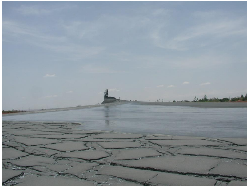
Figure 3.2: Paste tailings disposal towers located in the Bulyanhulu Mine tailings storage facility in October 2004 (picture taken by the Author).
