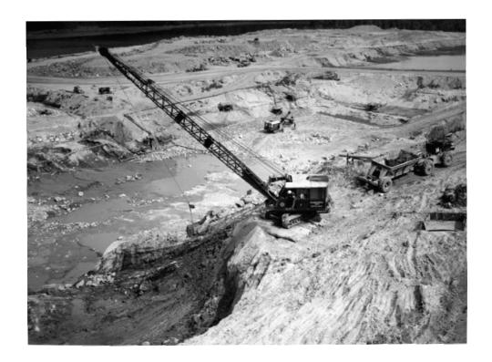
Figure 2-10: 1940 – Construction of Franklin Falls Dam, photograph taken looking downstream to stilling basin from west abutment, provided by Paul E. Cote and Pullen (2012).
