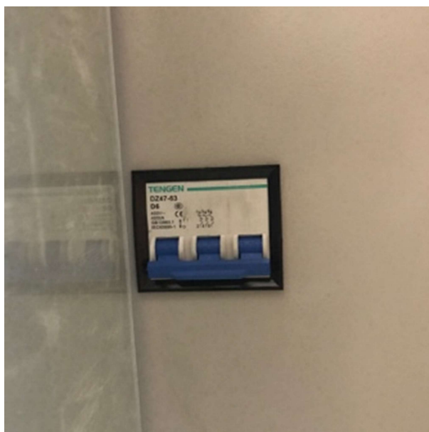
Figure 5 Braiding machine power breaker on the left side of the electrical box
