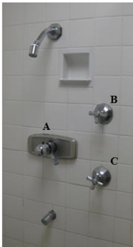
Figure A2.1: Photo of the faulty shower device in Wing 3. A: mixing valve, B: Upper shower faucet, C: Lower shower faucet. When the patient only closes the upper /lower shower faucet, hot and cold water constantly mix in the mixing valve.
