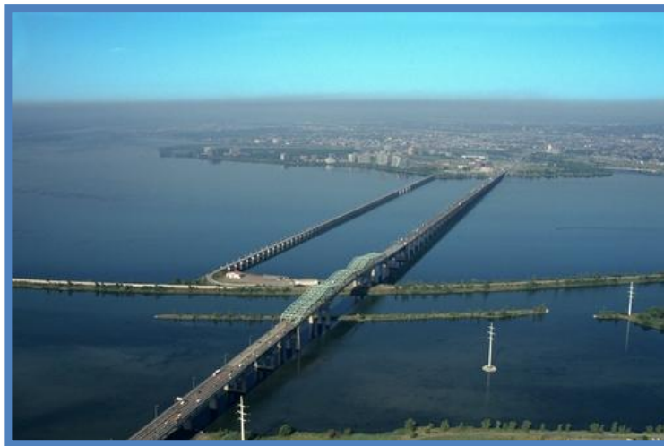
Figure 4.1: View for existing Champlain Bridge ( Ministry of Transports Quebec, 2011 )
