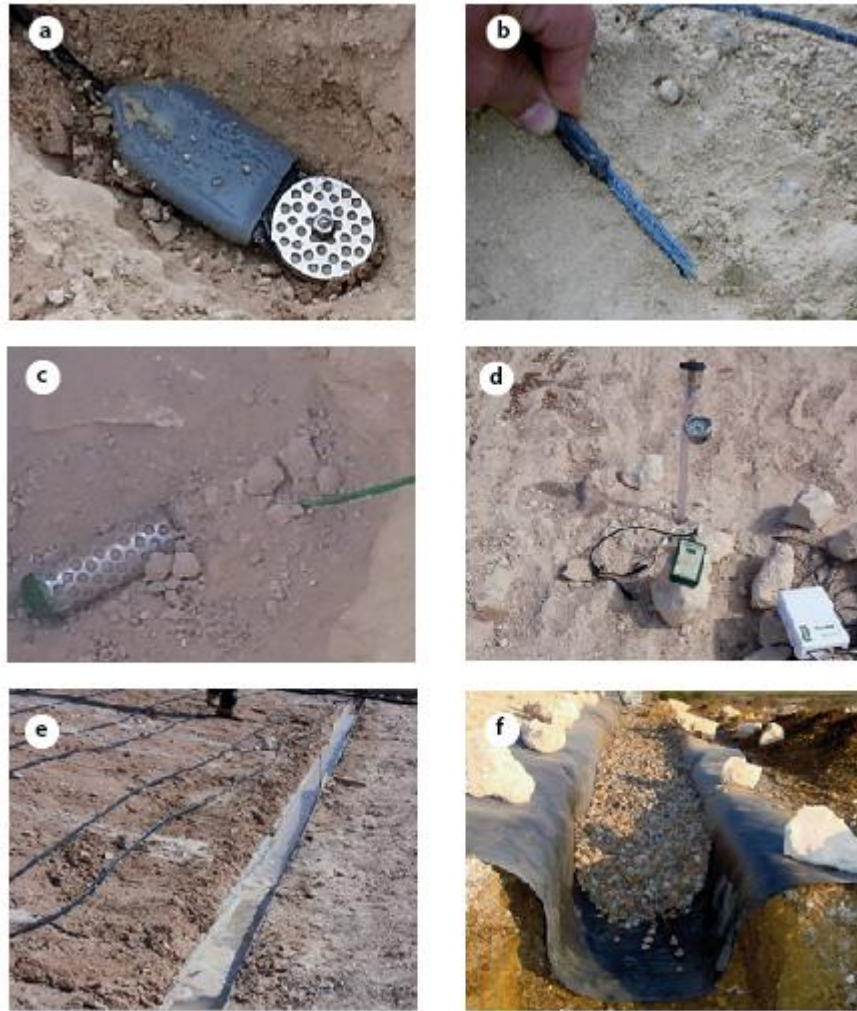
Figure 4.3: Photos illustrating the instrumentation used to monitor the inclined SR experimental cell (a) matric suction sensor (MPS-2) (b) volumetric water content sensors (EC5) (c) Matric suction sensor (Watermark) (d) JetFill tensiometer (e) surface runoff collector (f) later drainage collectors
