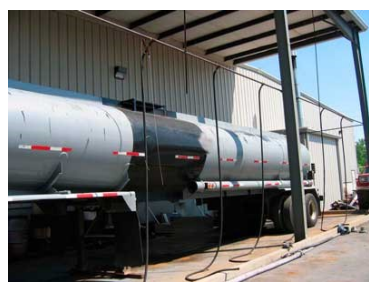
Figure 5-1 : Tanker wash facility (NIOSH, 2014)
