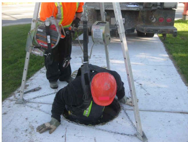
Figure 4-3 : Tripod and winches for fall protection and external rescue; wearing of a Class A harness
