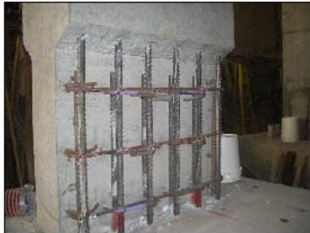
Figure 6.5 : Bar configuration and surface preparation in the repair zone
