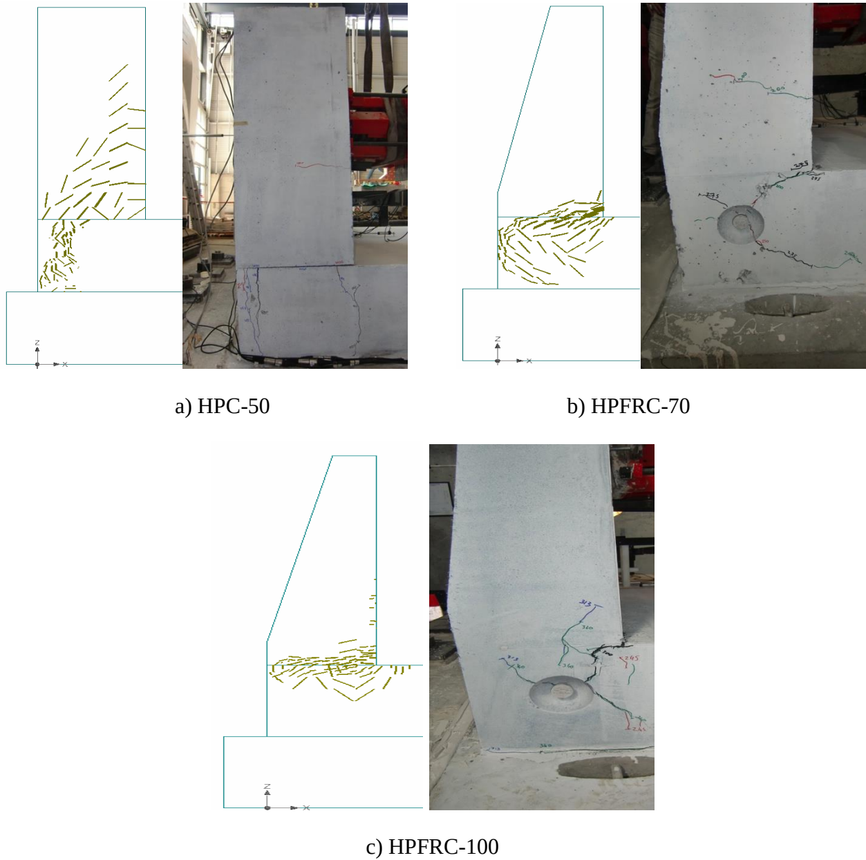
Figure 3-5: Experimental and numerical cracking pattern at ultimate load
