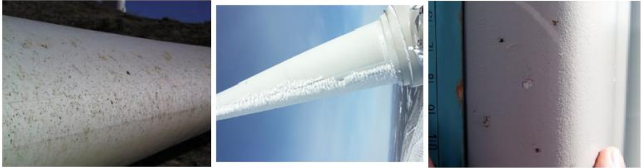
Figure 3-1 Rough surfaces of wind turbine blades caused by insects, ice, and erosion, respectively. (KellyAerospace) (Weiss) (BladeSmart)
