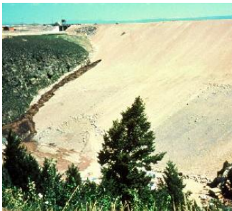
Fig. 3 : initiation of the failure
