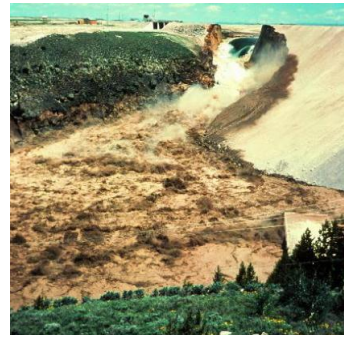
Fig. 5 : Failure of the Teton Dam Photography credit : Arthur G. Sylvestre
