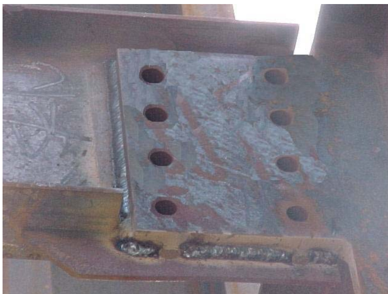
Figure 1-4 - Retrofit Weld on Shear Tab Connection (Photo: DPHV)
