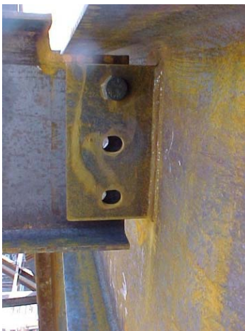
Figure 1-3 - Hole Misalignment in Shear Tab and Supported Beam Web (Photo: DPHV)
