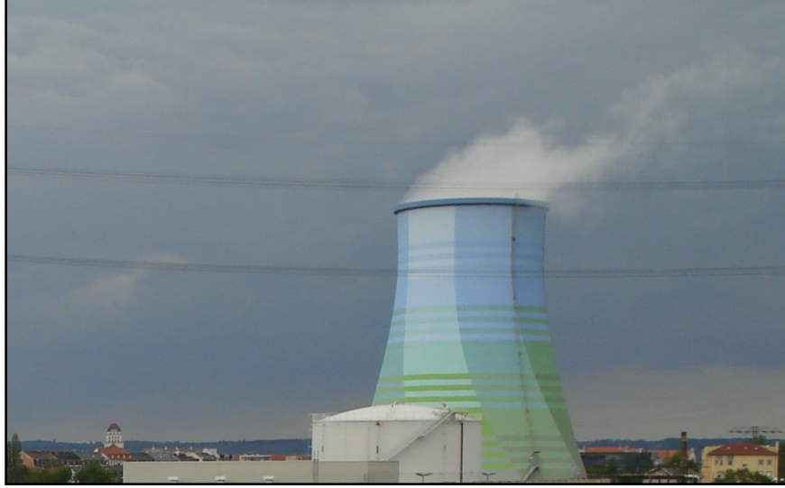
Figure 1.1 Example of a DCHX: in a cooling tower, the warm liquid mixes with ambient air. A portion of the water brings the air to saturation, and the rest goes in a container at the bottom of the cooling tower (cooling tower in Dresden, Germany)
