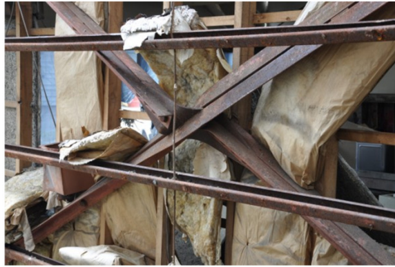
Figure 58. Lateral torsional buckling of the double angle steel braces due to thin gusset plates (3-story office building)
