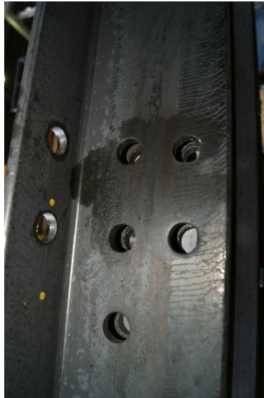
Figure 3.53: Retrofitted connection preparation
