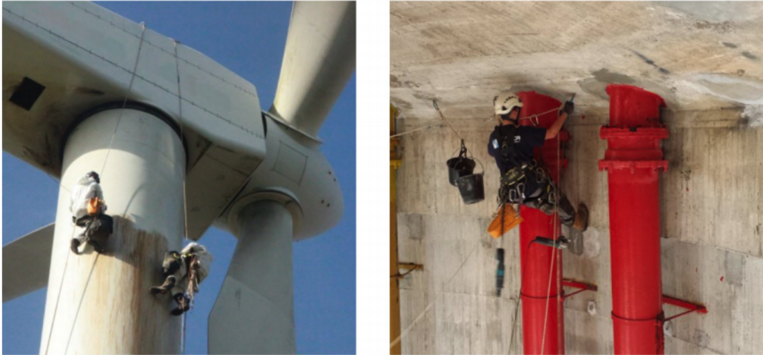
FIGURE 4.1 Examples of tasks performed by rope access technicians (wind turbine maintenance on the left, NDT of water pipes on the right), courtesy of Vertica (Brittany, France)
