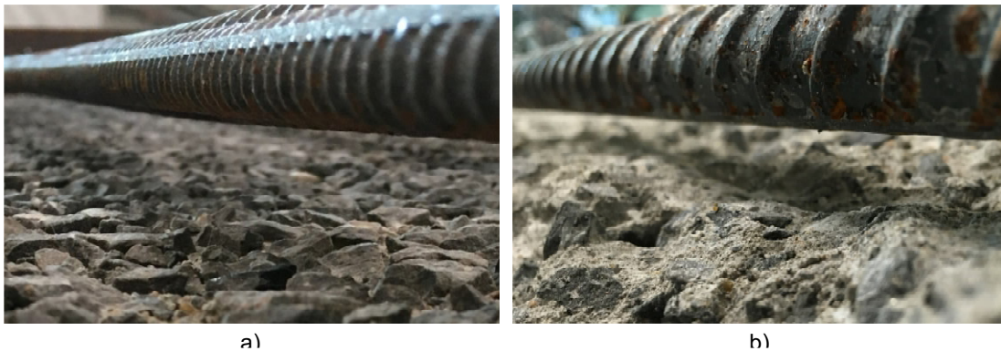
Figure 5-4 NSC-UHPC interface, a) obtained by a surface retarder for UD slabs, b) obtained by hydrodemolition for PD slabs
