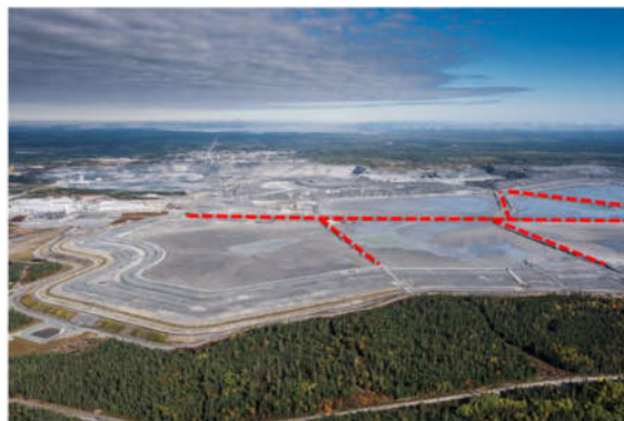
Figure 2-2: Malartic mine tailings impoundment with WRIs (Quebec, Canada). WRIs (shown with red dashed lines) are around 12 m wide and divide the impoundment into several compartments (IRME, 2019).
