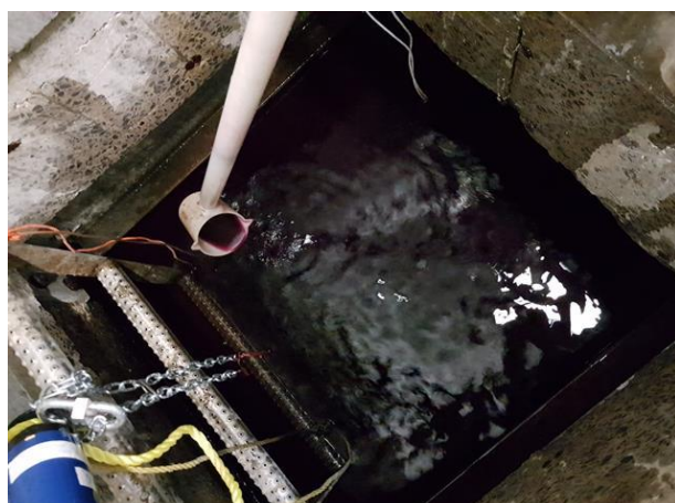
Figure 3-2 On-site oxidation using \text{KMnO}_4 in the sludge holding tank
